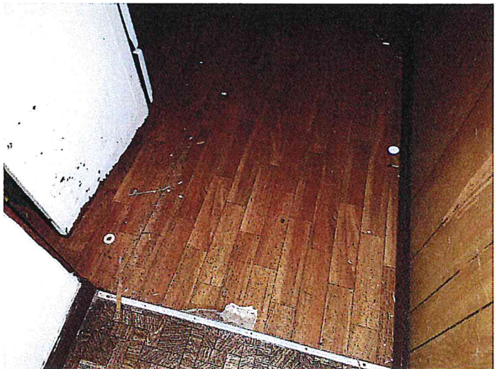
4/19/2016 SAMPLES S23 & S24 - VINYL SHEET FLOOR BOARD PATTERN Pic (16).jpg
