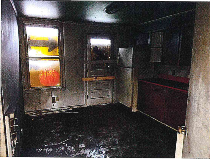
4/19/2016 517 A&B - INTERIOR A SIDE Pic (07).jpg
