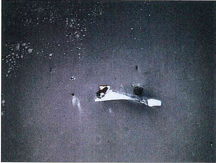
4/19/2016 SAMPLES S17 & S18 - GYPSUM BOARD WALL Pic (13).jpg
