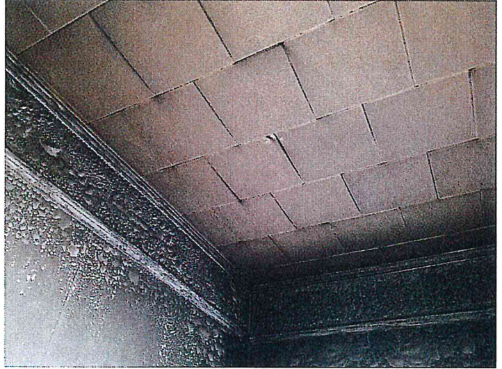
4/19/2016 SAMPLES S19 & S20 - 12X12 CEILING TILE WHITE - NAILED ON Pic (14).jpg
