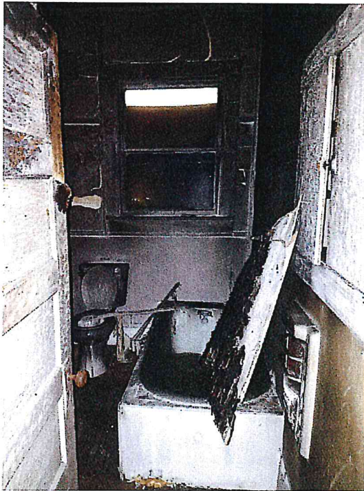
4/19/2016 517 A&B - INTERIOR A SIDE Pic (05).jpg
