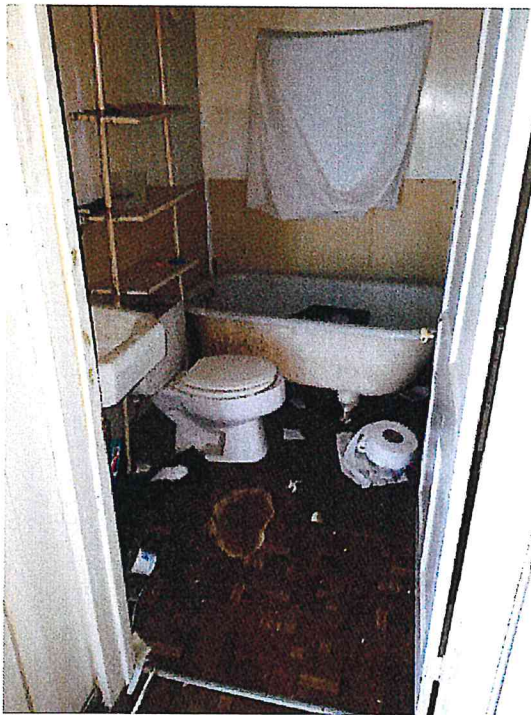
4/19/2016 517 A&B - INTERIOR B SIDE Pic (09).jpg
